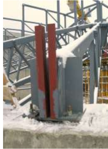
Fig. 7 A support joint of the semi-truss during erection of the cupola
