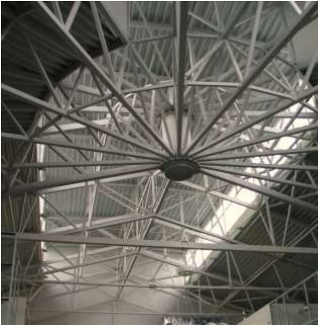
Fig. 6 A view of the central vertical braces
