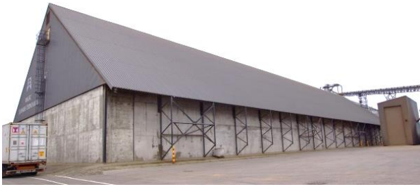
Fig 4 An outside view of the storage facility
