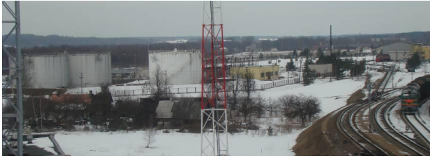
Fig. 5 The areal view on the diesel fuel tanks exposed to the danger of a potential BLEVE on rail (authors' photo)
