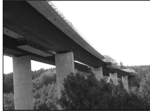
Fig. 1 Border Bridge on D8 highway
