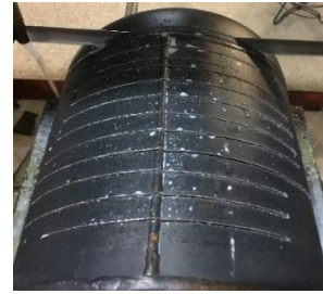
Fig. 20 Cutting operation of new tank
